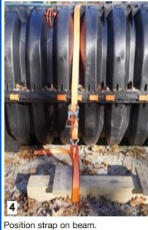
Position strap on beam.
