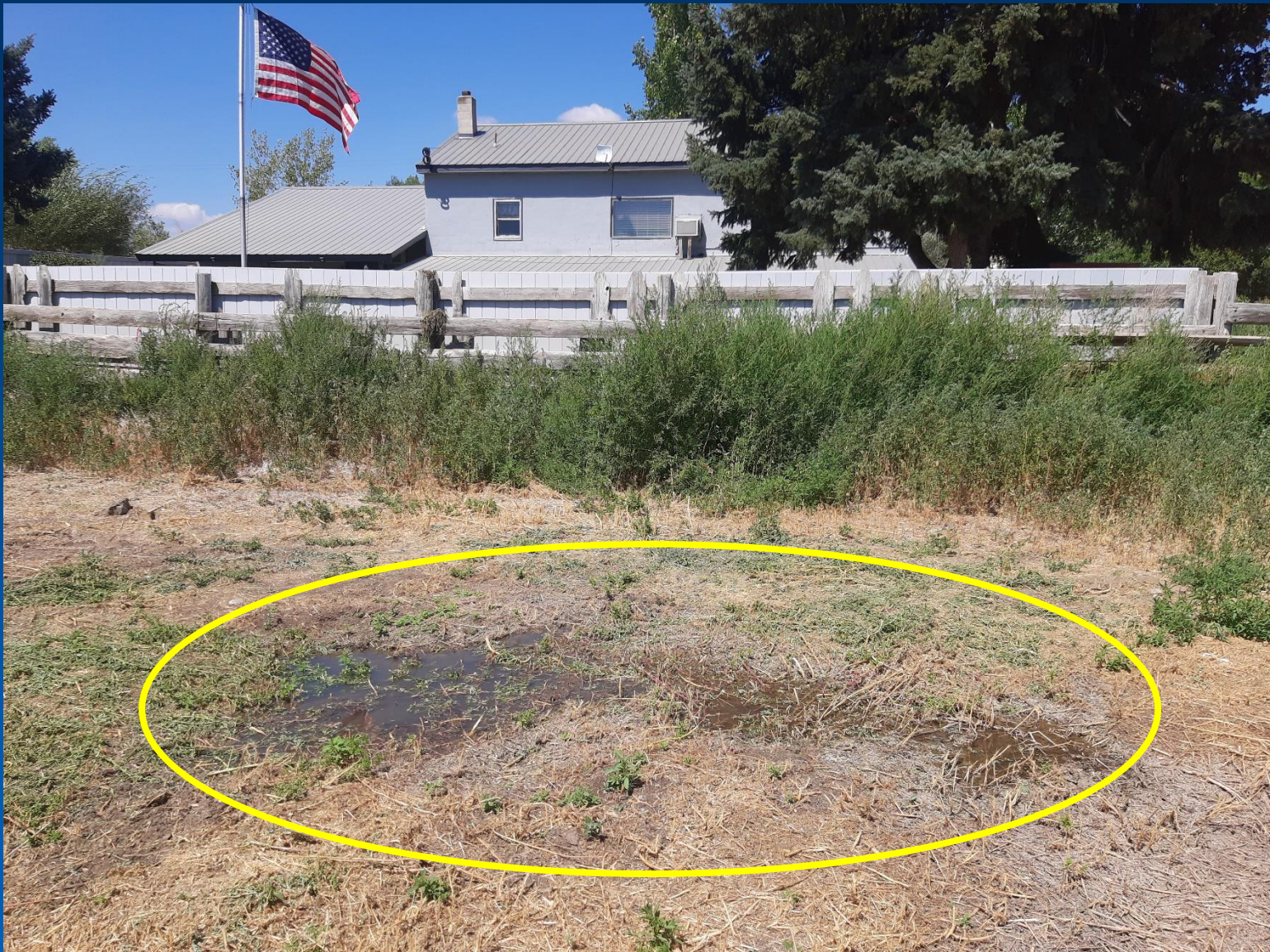
Surfacing of sewage in a failed system.
